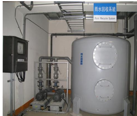
↑ Factories installed with
