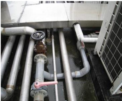
↑ Factory Rain water recycling system
