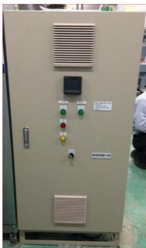
Elevator installed with energy-saving control devices.
